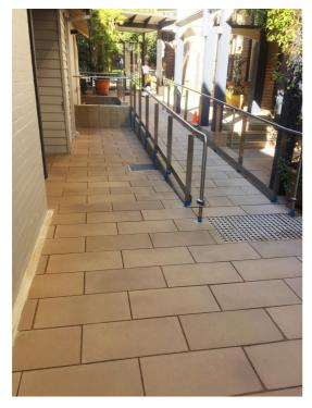
Simon and his team cleaned the new concrete pavers thoroughly and left it to dry. Once it was completely dry, the sealer was applied.
